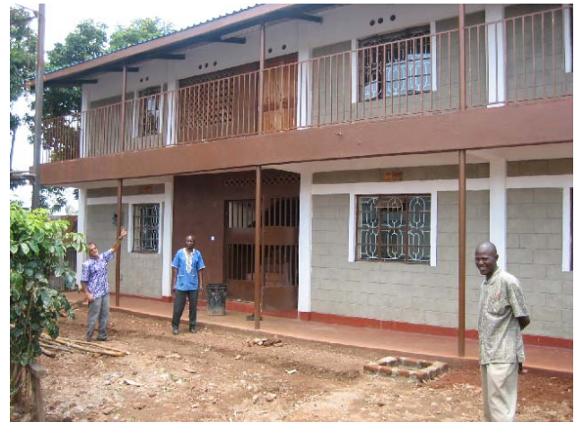
The new dormitory nearing completion in September 2007
