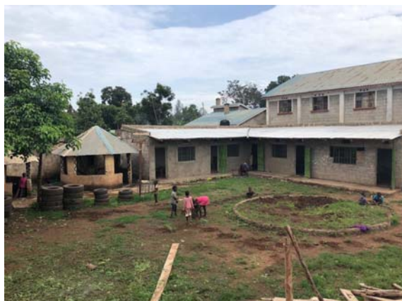
New primary school compound
